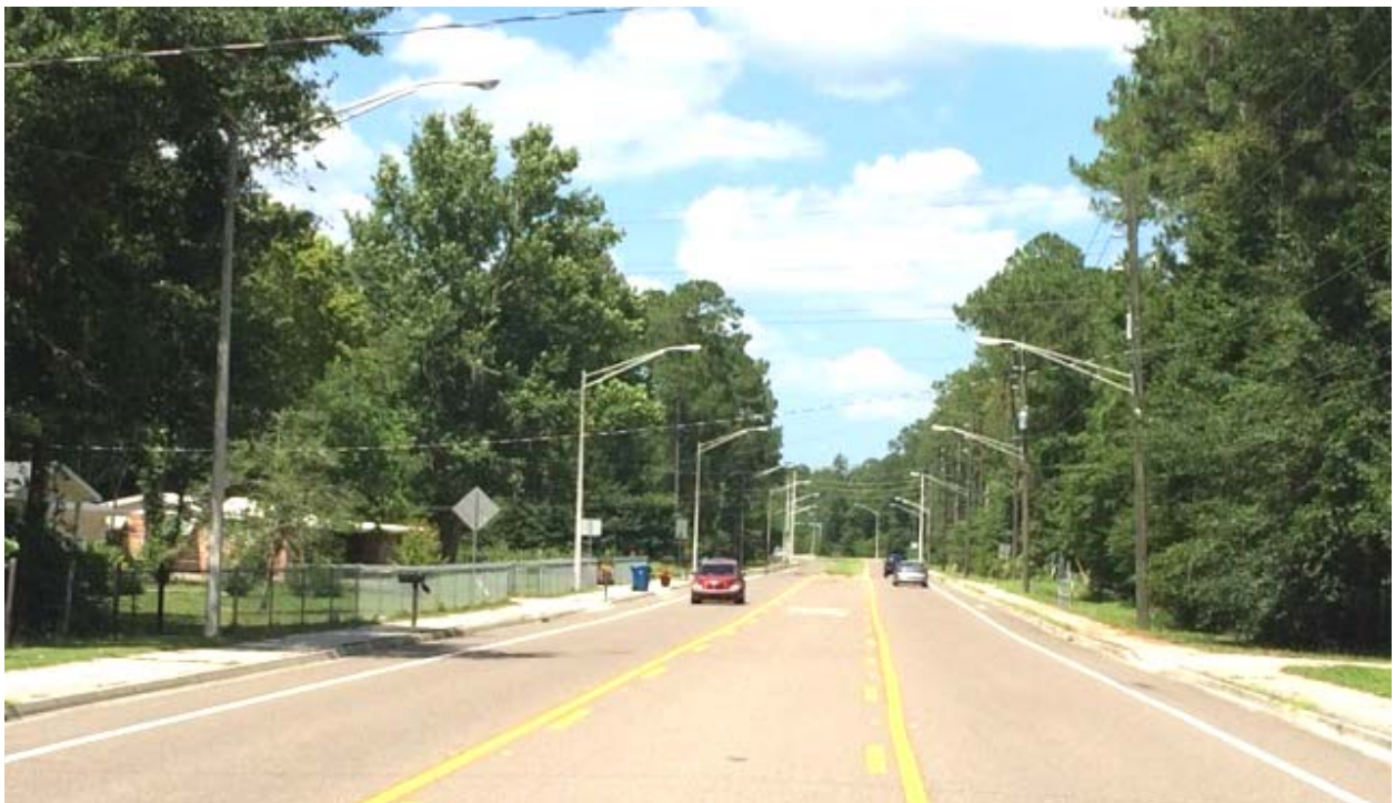
The subject site ahead on the left facing northeast along Starratt Rd.
